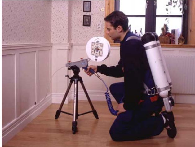
Figure 7 Fiber blowing from apartment
