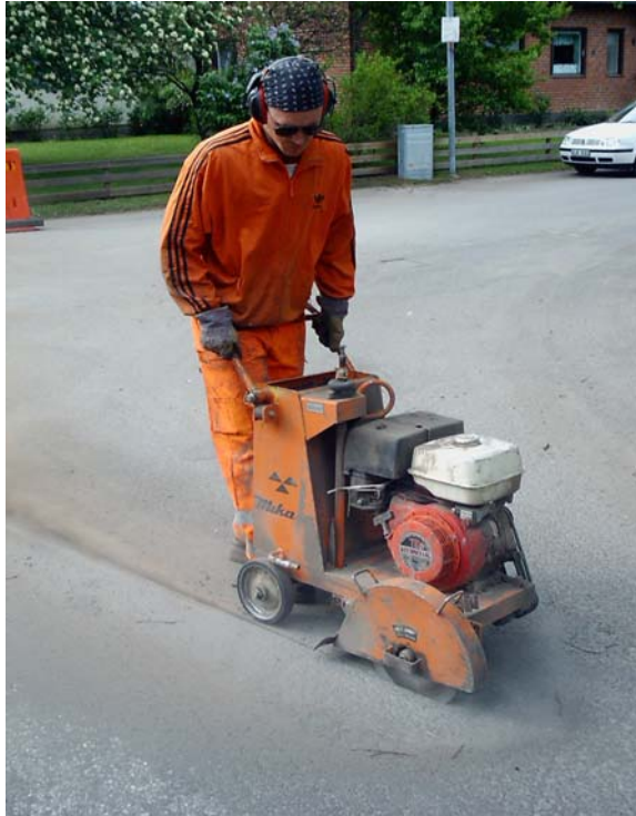
Figure 4: Micro trenching on the pavement
